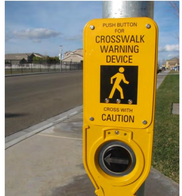
*Top and Above* An in-pavement lighted crosswalk and a push button to activate the warning sign.
