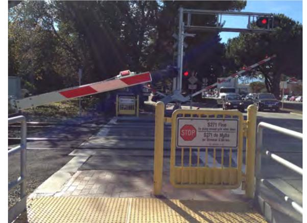
*Detectable warning surfaces and pedestrian gates placed on sidewalk approaching railroad tracks*
