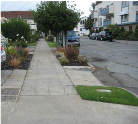
*Optimal driveway design provides a smooth and continuous sidewalk with the driveway apron at the street edge within the planting strip*
