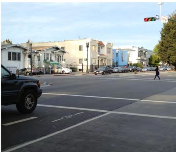
*A bicycle detector loop with a pavement marking at a signalized intersection. When the detector senses the bicyclist, it changes traffic lights from red to green.*
