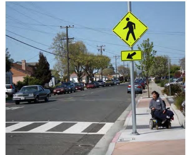
*An ADA-compliant curb ramp should be provided at each end of the crosswalk.*
