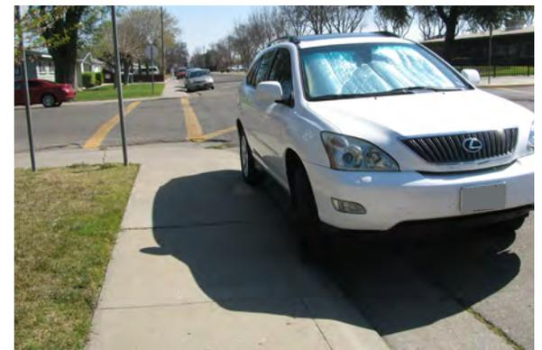
*A car parked on the sidewalk due to a rolled-edge curb.*
